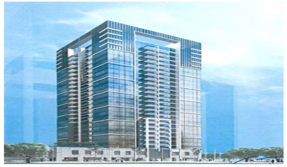
CAPITAL CITY CENTRE, ADNEC – ABU DHABI Supply, Installation, Testing & Commissioning of CCTV, Gate Barrier and Structure Cabling – Completed Consultant: AMAR Golden Design
