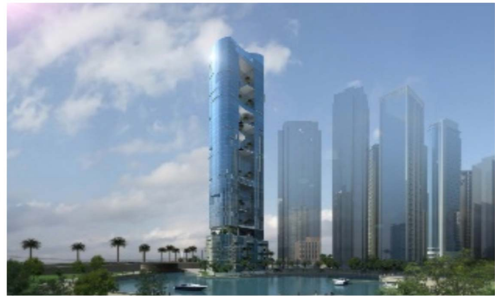
SARAYA TOWER – ABU DHABI Design, supply, installation, testing and commissioning of CCTV System and Structured Cabling Ongoing project, ABU DHABI
