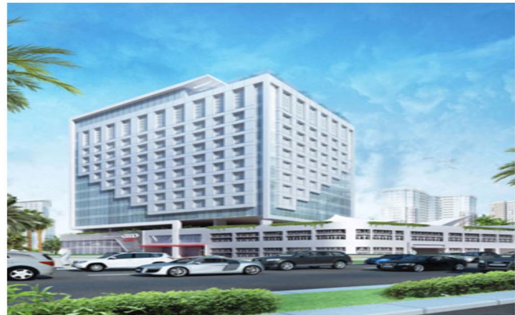
C40 (AUDI SHOWROOM BUILDING) Supply, installation, testing and commissioning of CCTV, Access Control System and Structured Cabling 2015-2016, ABU DHABI
