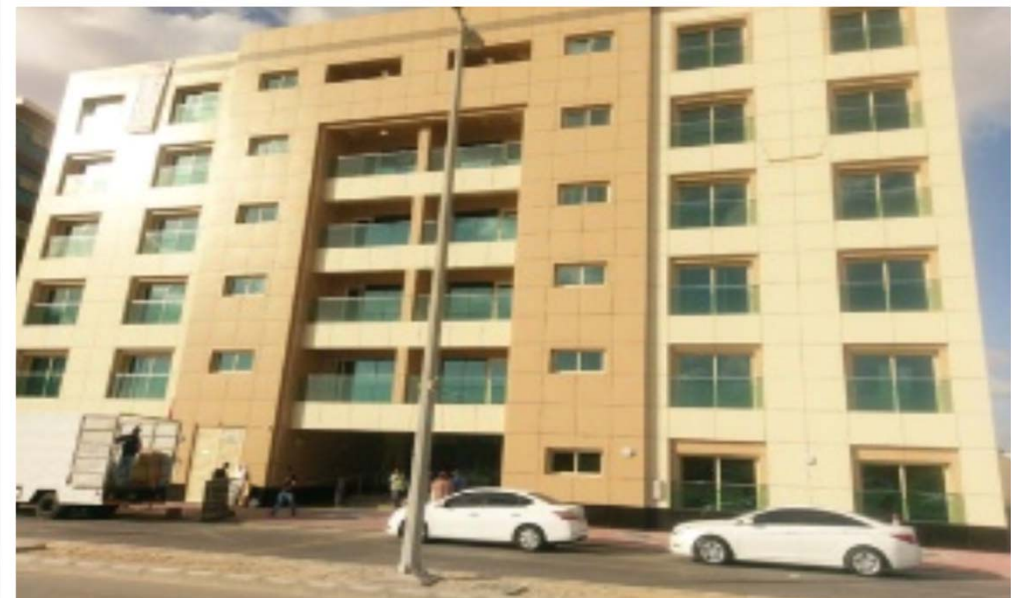
RESIDENTIAL PROJECT in RAWDHAT C104 & C105 ABU DHABI Supply of CCTV System - 2016 Consultant: Rabros/ UTT
