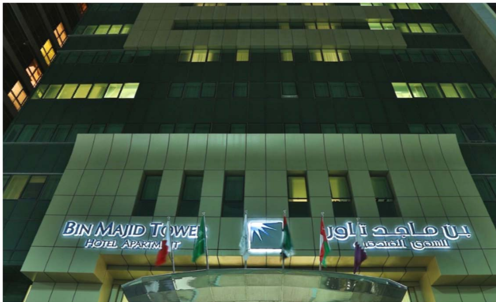
BIN MAJID TOWER, HOTEL APARTMENT – ABU DHABI Supply of CCTV System - 2013 Client: RTS
