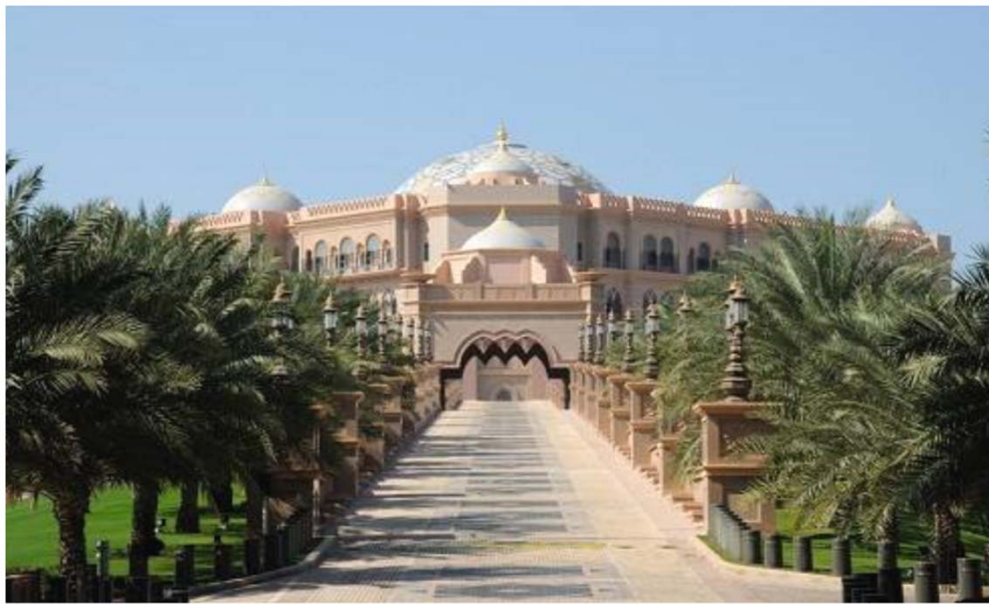
PRIVATE VILLA, SEA PALACE – ABU DHABI CCTV System, Home Automation, light Control, Access Control and Security System Design - September 2014 Consultant: H.H. TBZ/ Bainona Consulting
