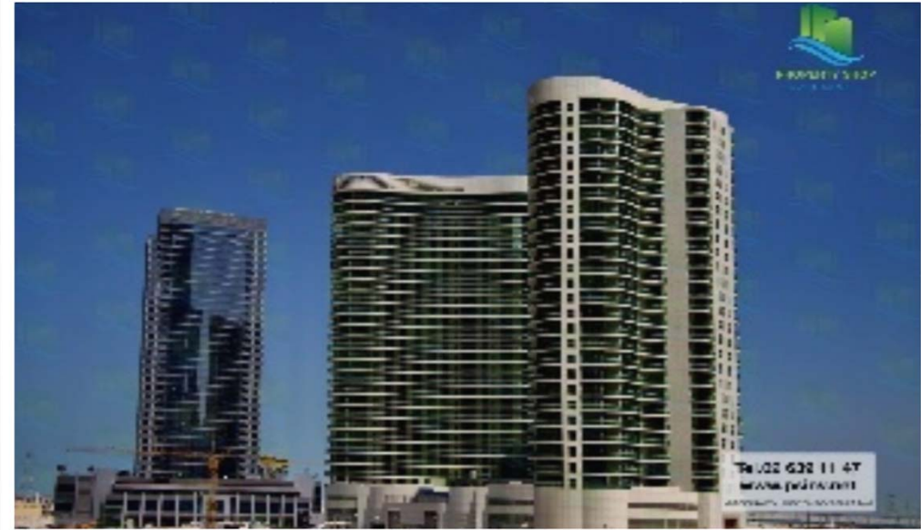
M RESIDENTIAL TOWER, Reem Island - ABU DHABI Supply, installation, testing and commissioning of Home Security System - Ongoing Client: Rabros / UTT
