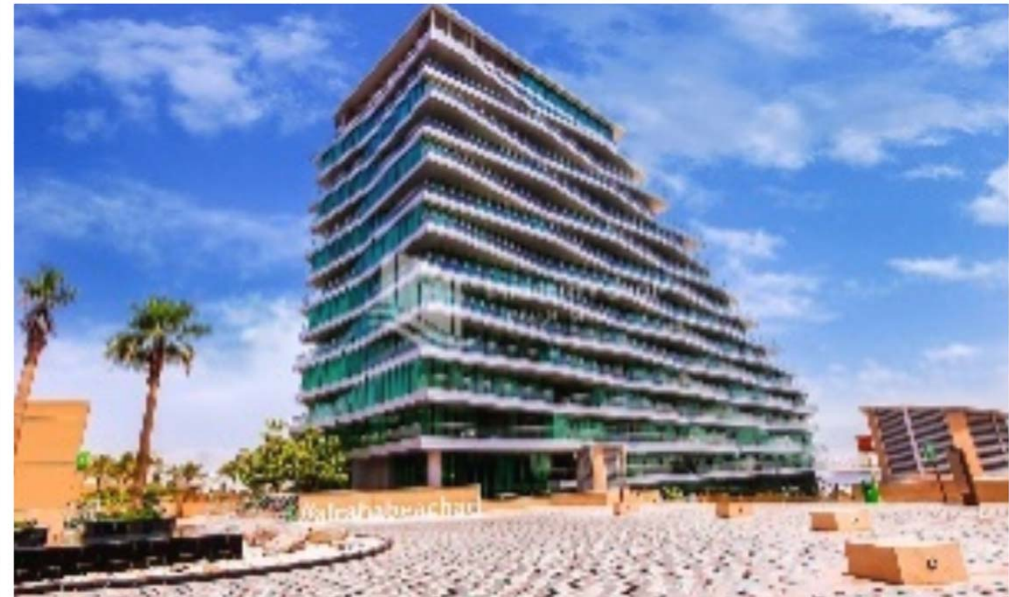
AL RAHA COMMERCIAL TOWER - ABU DHABI Supply & Installation for ELV system ( SMATV , SCS , CCTV , Intercom , Access Control & Gate Barrier ) – May 2019 Client: Al Dyar / Gulf Coast
