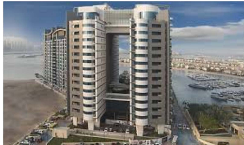
OCEANA HOTEL & APARTMENTS - DUBAI Supply, installation, testing and commissioning of Access Control System and Structured Cabling - Ongoing Client: DRC / Seven Tides LLC
