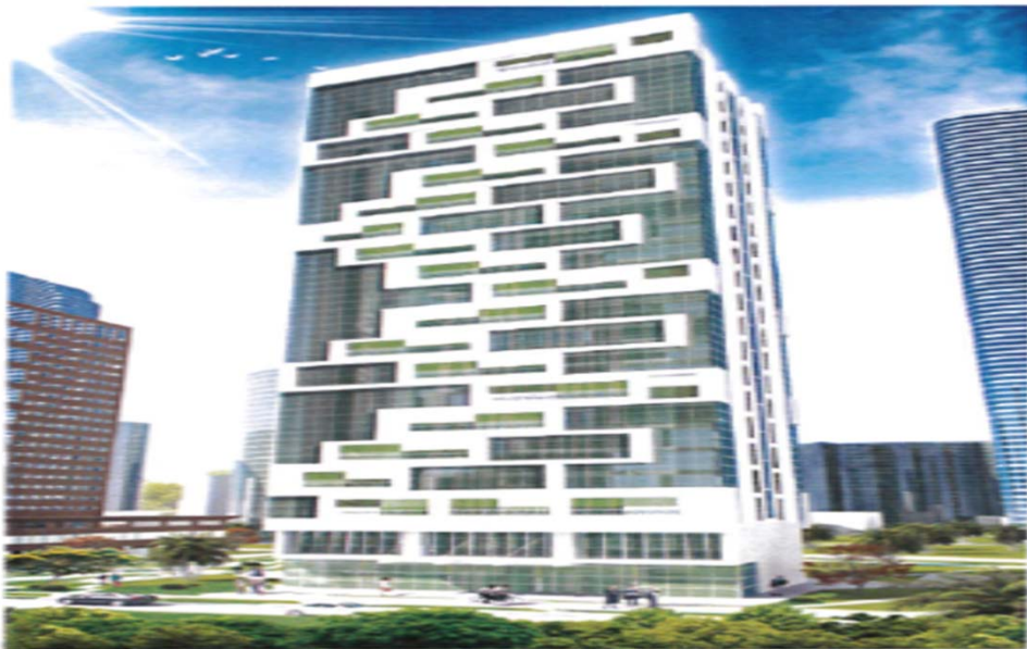
LULU TOWER – ABU DHABI Supply & Installation for ELV system ( SMATV , SCS , CCTV , Intercom ) – May 2019 Client: Ghantoot / Ecotherm
