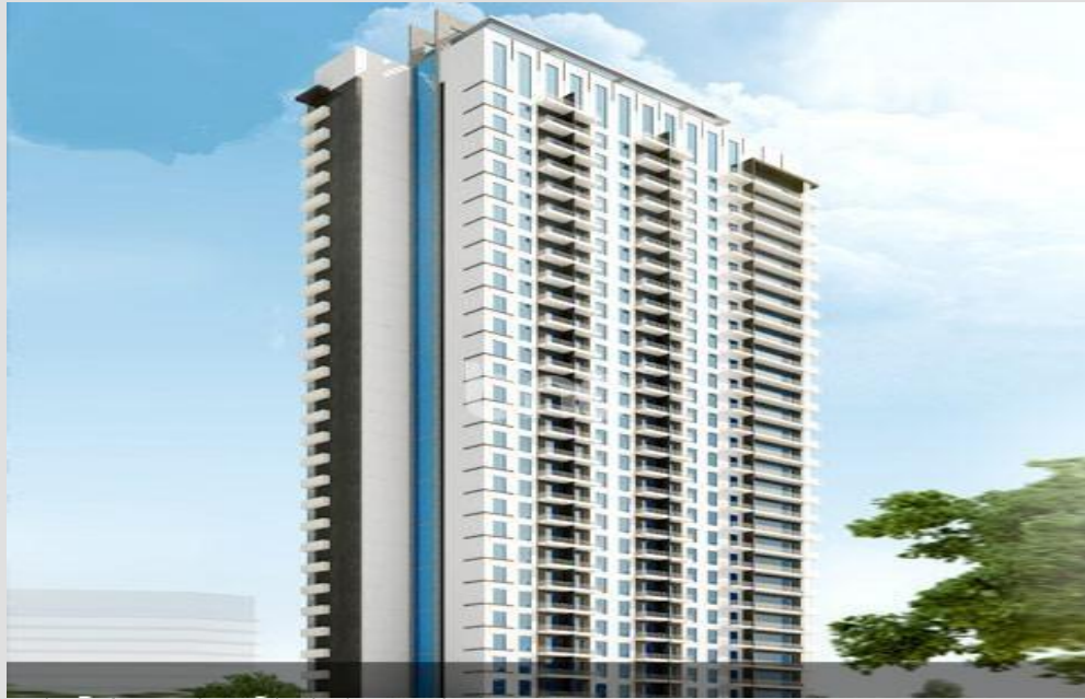
AZURE TOWER – ABU DHABI Supply, Installation, Testing & Commissioning of CCTV, Access Control System- 2018
