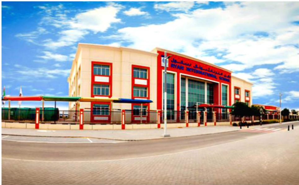
RAYAN INTERNATIONAL SCHOOL– ABU DHABI Supply, installation , testing and commissioning for CCTV System and Structured Cabling - September 2015
