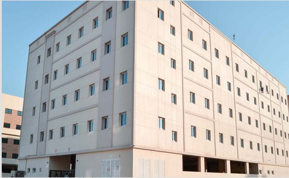
LABOUR CAMP – DUBAI Supply, Installation, Testing & Commissioning of SMATV and Structure Cabling 2018
