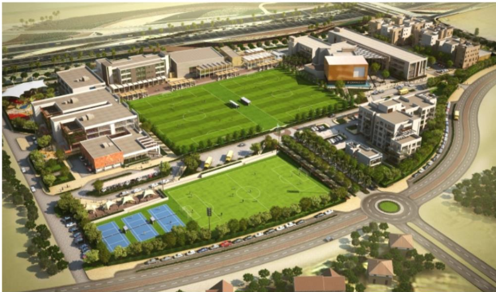
Cranleigh School, Saadiyat Island – ABU DHABI Supply of CCTV System Client: AECOM
