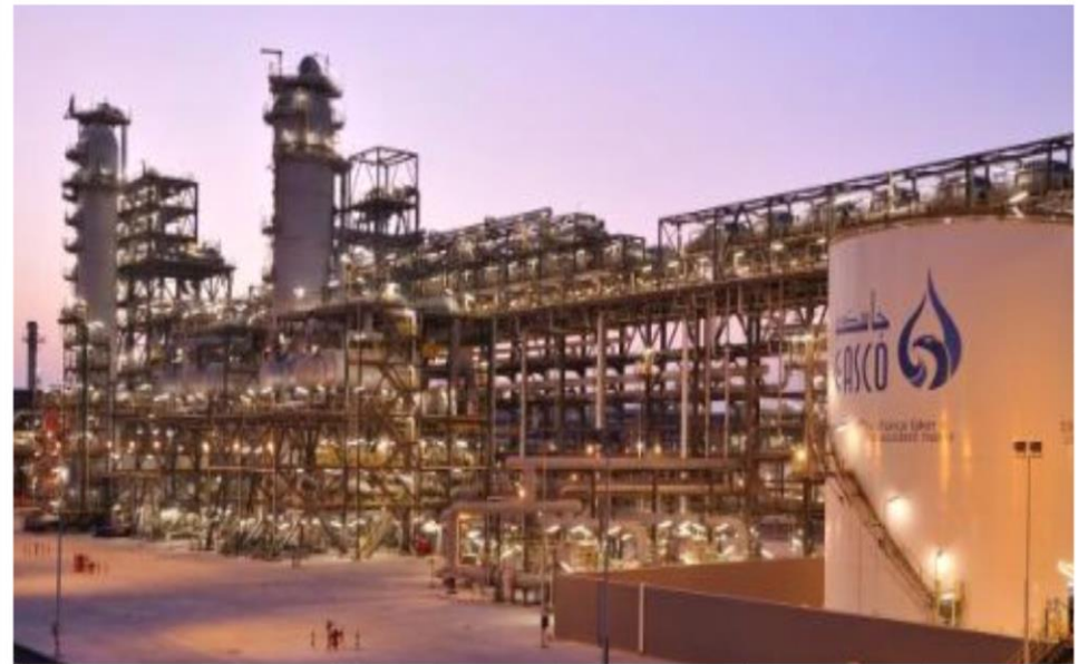
GASCO– ABU DHABI Supply, installation, testing and commissioning of active components, Telephony System and Structured Cabling September 2015
