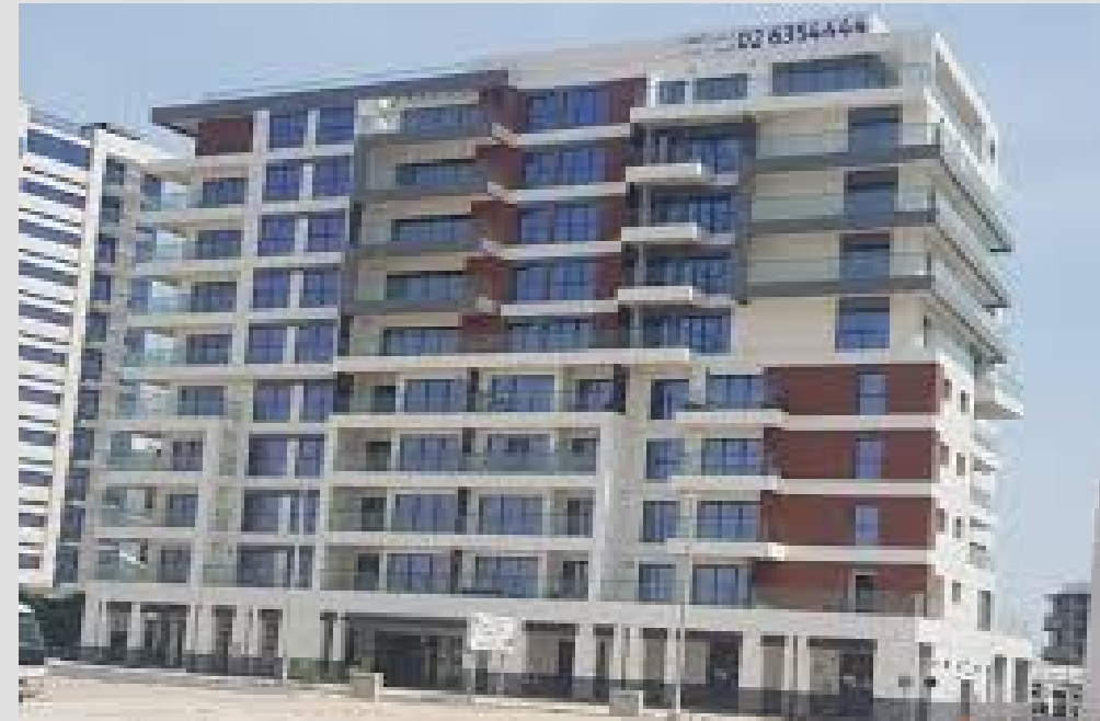
SHAIKHA WADEEMA, C9, C10 – ABU DHABI Supply, installation, testing and commissioning of Gate Barrier – September 2018 Consultant: World Planners Consultants Engineer
