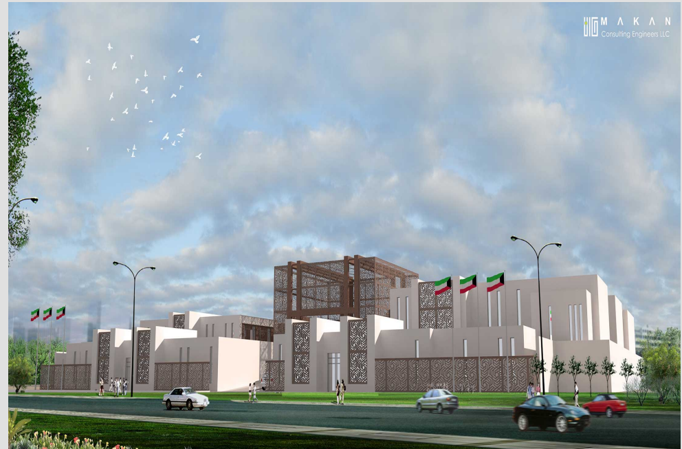
Embassy of state of Al Kuwait – ABU DHABI Supply, installation, testing and commissioning SCS, CCTV, ACS, AV, Q-management, Active component, Intercom, UPS, IPTV Systems 2023
