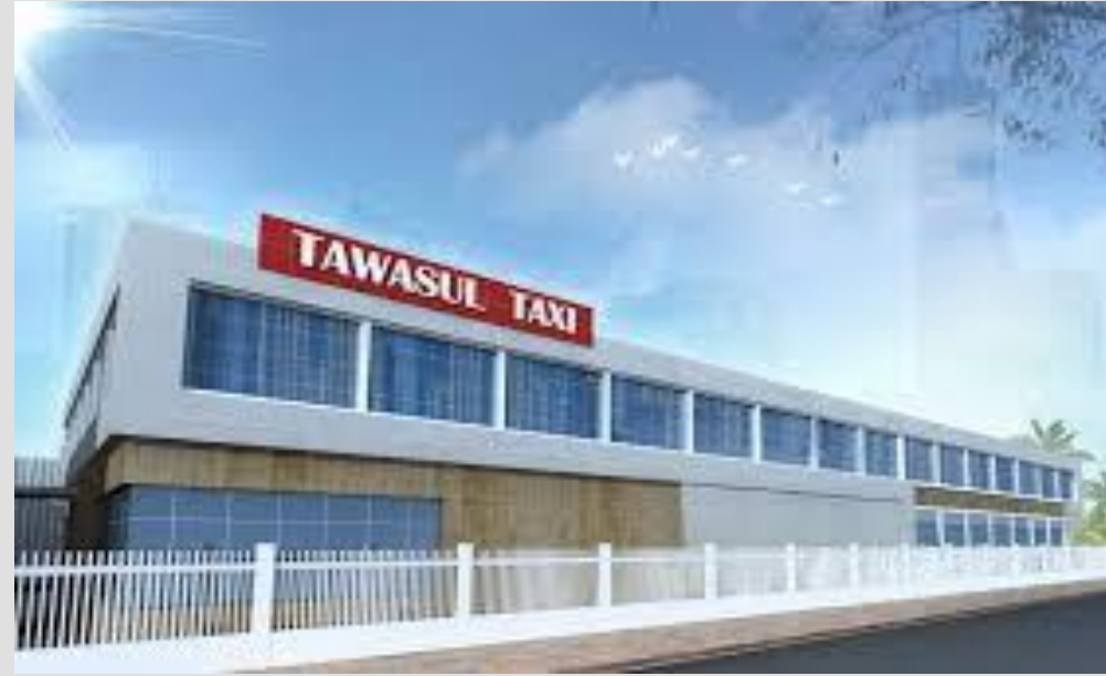
TAWASUL TAXI – ABU DHABI Supply, installation, testing and commissioning of CCTV and Structure Cabling – 2017 Consultant: Bainona Engineering Consultancy
