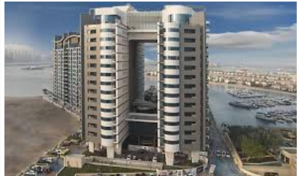
OCEANA HOTEL & APARTMENTS - DUBAI Supply, installation, testing and commissioning of Access Control System and Structured Cabling - 2016 Client: DRC / Seven Tides LLC
