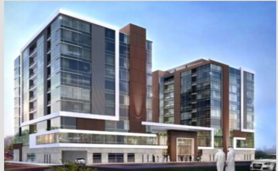
AIZEBAQ COMMERCIAL BUILDING – ABUDHABI Supply, Installation, Testing & Commissioning of SCS,ACS,CCTV,INTERCOM,GB 2023
