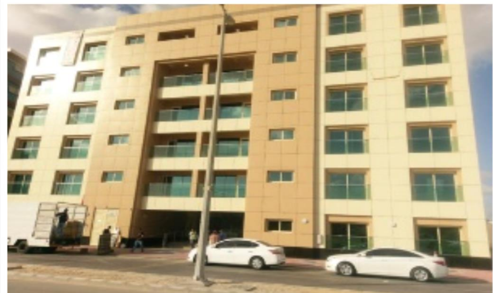
RESIDENTIAL PROJECT in RAWDHAT C104 & C105 ABU DHABI
