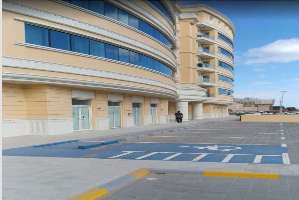
AL NAHYAN COMMERCIAL BUILDING – AUH Supply, Installation, Testing & Commissioning of CCTV, Structure Cabling, SMATV and Video Intercom System 2019 Consultant: Golden Planne Consultants
