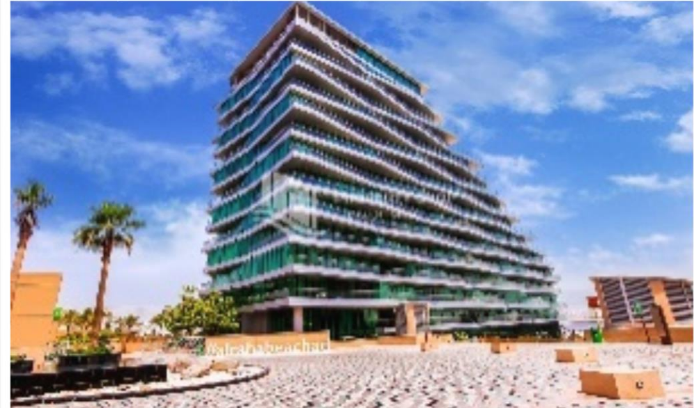
AL RAHA COMMERCIAL TOWER - ABU DHABI Supply & Installation for ELV system ( SMATV , SCS , CCTV , Intercom , Access Control & Gate Barrier ) – May 2019 Client: Al Dyiar / Gulf Coast
